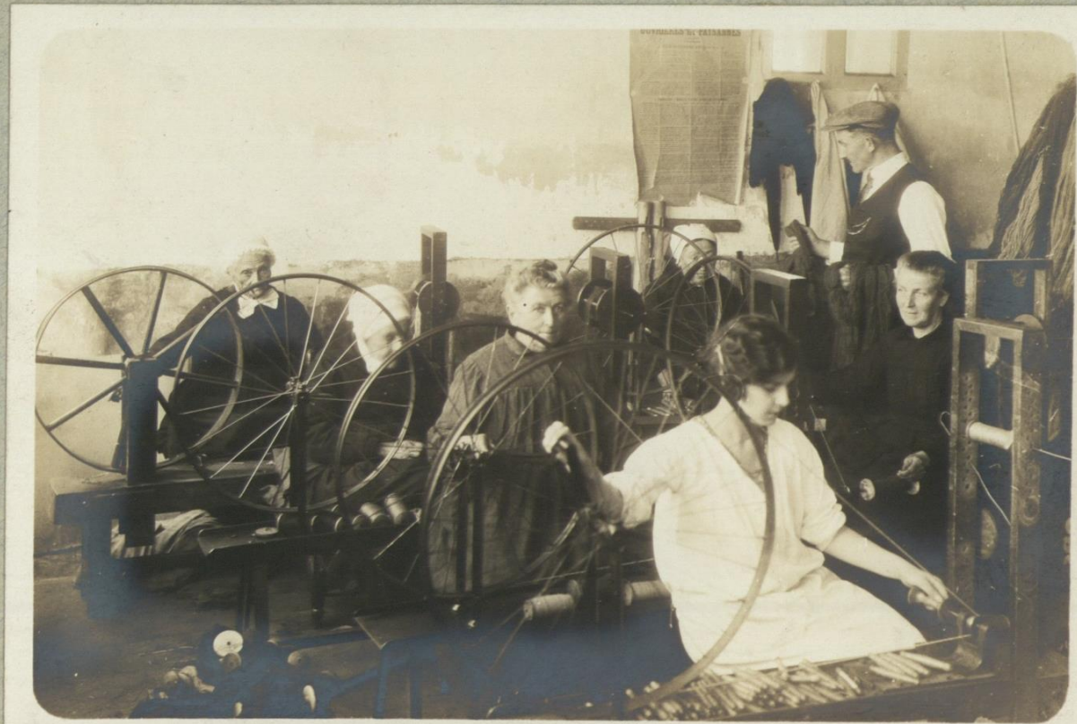
3° Aubusson Mills - Winders"Corner.
